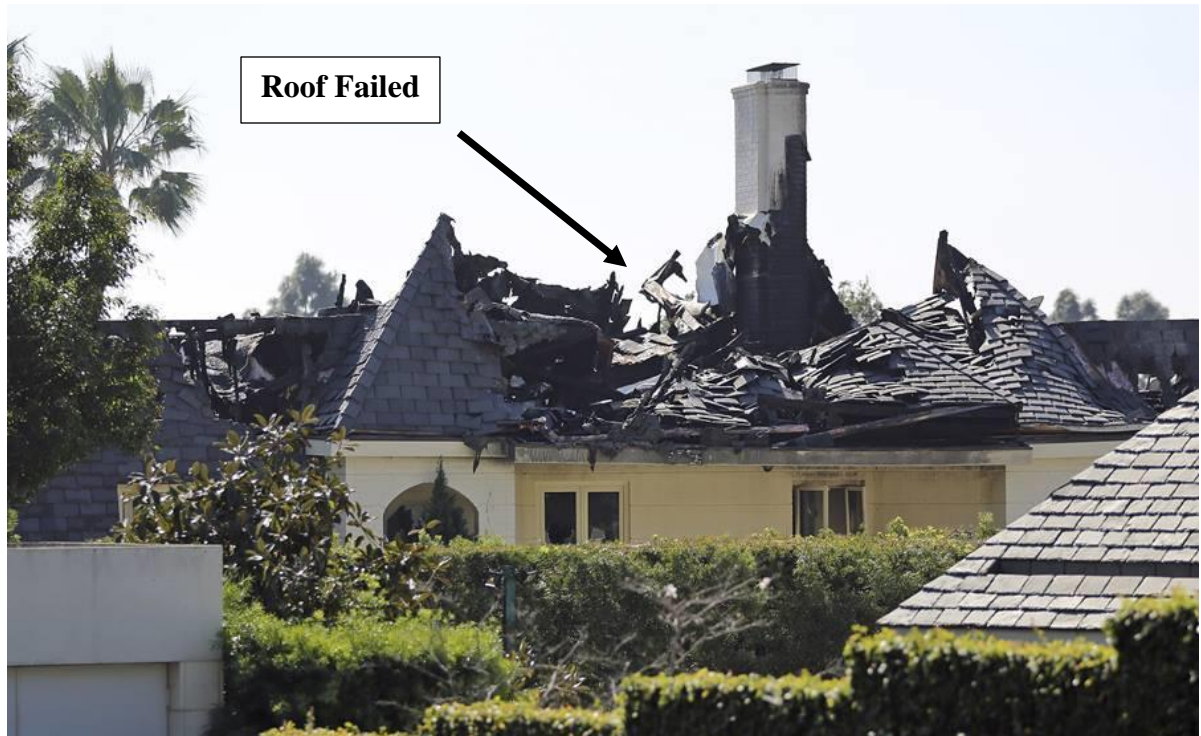
Figure 6 House Fire and Roof Failure (Human Made Disaster)
