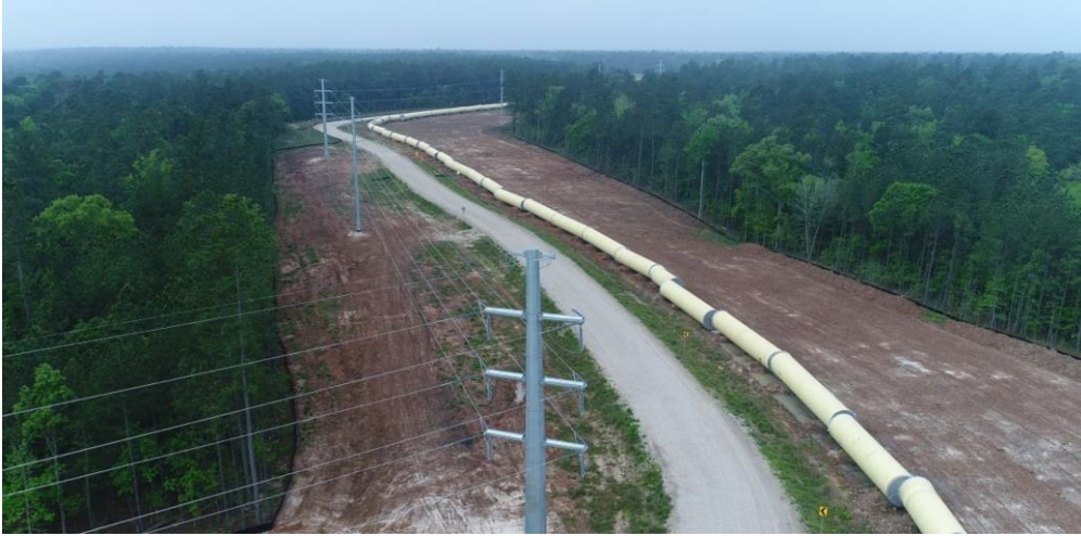
Dual 96-Inch Pipelines
