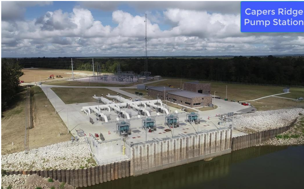
Capers Ridge Pump Station
