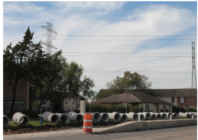
Beechnut Reconstruction Project
