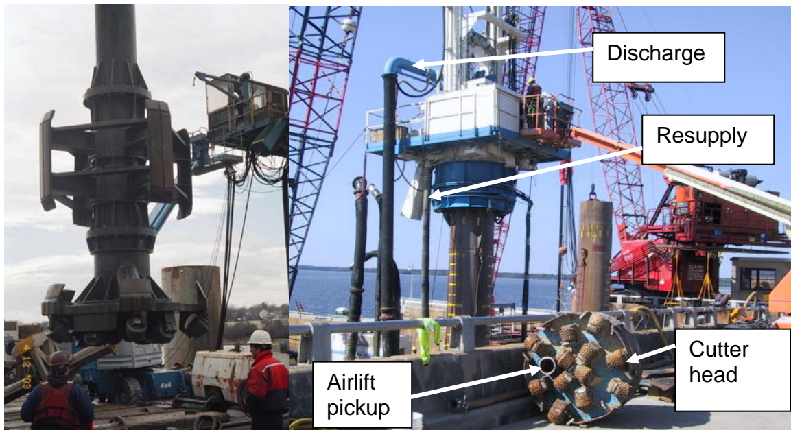
Figure 3 Reverse Circulation Drilling Equipment
