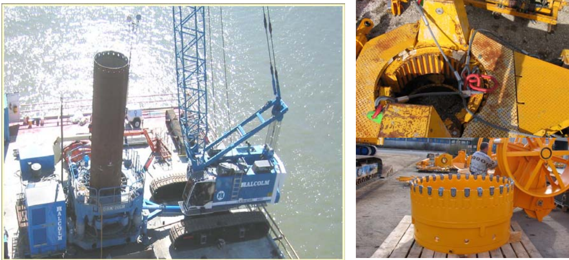
Figure 2 Oscillator Equipment for Installation of Segmental Casing
