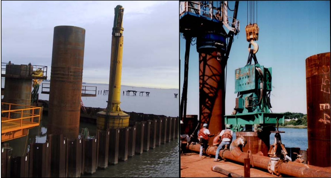
Figure 1 Installation of Permanent Casing
