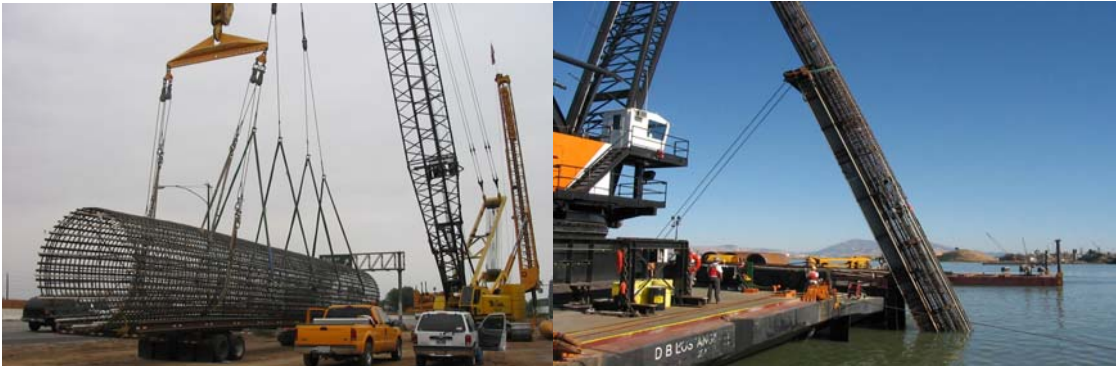
Figure 5 Lifting of Large Reinforcing Cages
